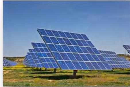
Solar energy includes solar water and space heating as well as taking solar photovoltaic panels to convert the sun's rays into electricity. Solar panels can typically produce between 120 and 200 watts per square meter at an installed cost of \$11 to \$22 per watt, according to the American Solar Energy Society but these costs are becoming less every year as more solar units are commissioned and new more cost effective technologies are developed.
